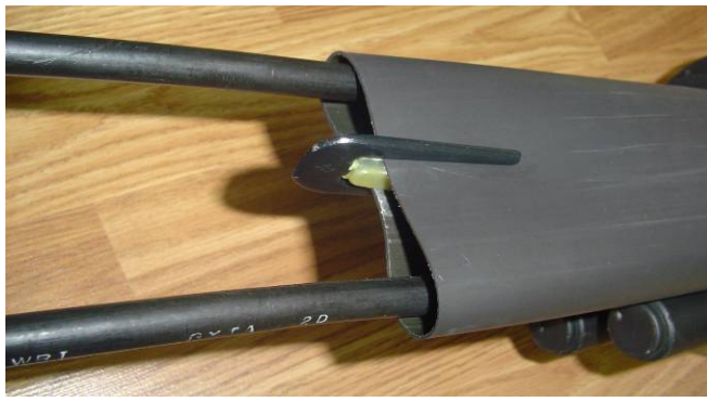
(14) Usage of branch folk: when heating the oval entry port, folk the heat-shrinkable tube to separate the two cables and heat-shrink it follow the steps above.
