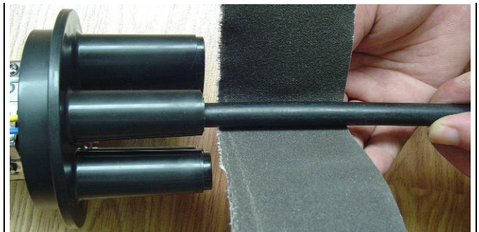
(11) Sand the cable and entry ports that need to heat-shrink by abrasive paper. Wipe the dust that be left after sanding away.
